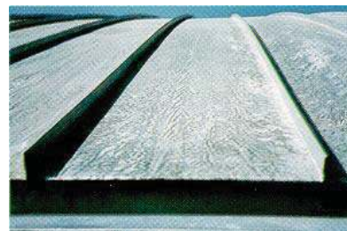
Figure 3. Stain on a GALVALUME ® roof panel under strippable coating.
